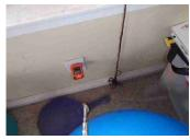
The room has one register and given its size two would be normally required which you should be aware of. The room will be colder than the rest of the home due to this condition.
