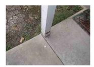
There is exposed electrical wiring on the corner of the structure that should terminate in a sealed junction box.
