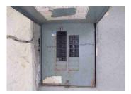
A 40 amp breaker is double tapped with a 20 amp wires which is a fire hazard and should be servcied by an electrician.
