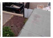
The roof to wall transition is not metal and the roll roofing has detached from the home which needs servcied
