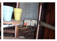
The outlet on the interior wall is recessed in the wall and needs to be servcied to be functional.
