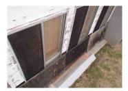
There is water damage to the eves and sheathing that is visible under the eves which needs serviced.
