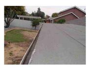
The roof only has partial gutters and full gutters are recommended for the general welfare of the residence and its foundation, inasmuch as moisture is a perennial problem on any property which can lead to settling and cracking of the foundation stem walls.
